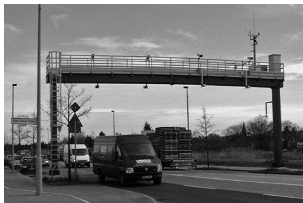
Figure 9 Experimentation road at DLR Berlin for the system tests
